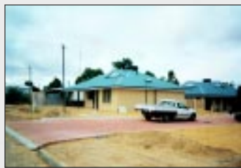
New houses being built in the Shire of Victoria Plains.
